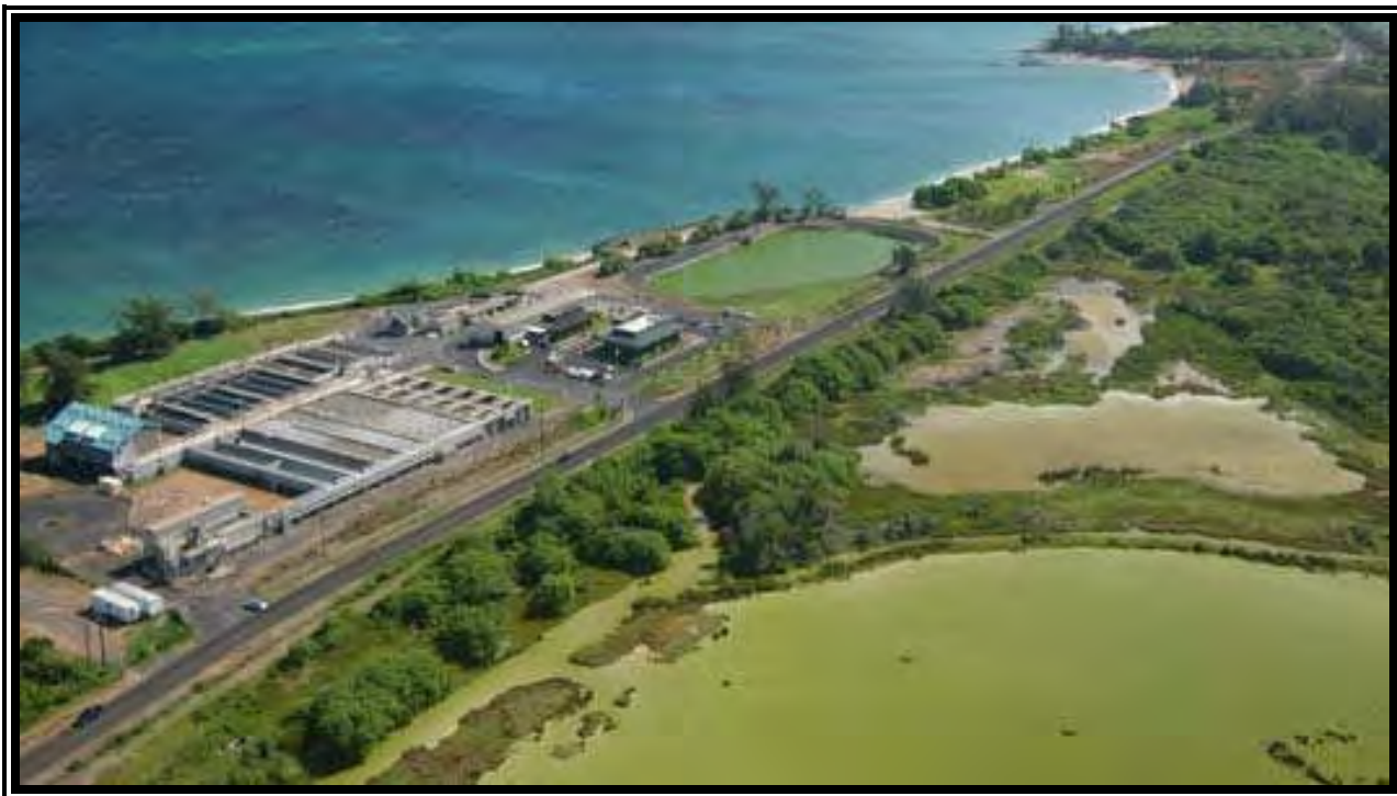
Central Maui Wastewater Reclamation Facility, Kanahā.
