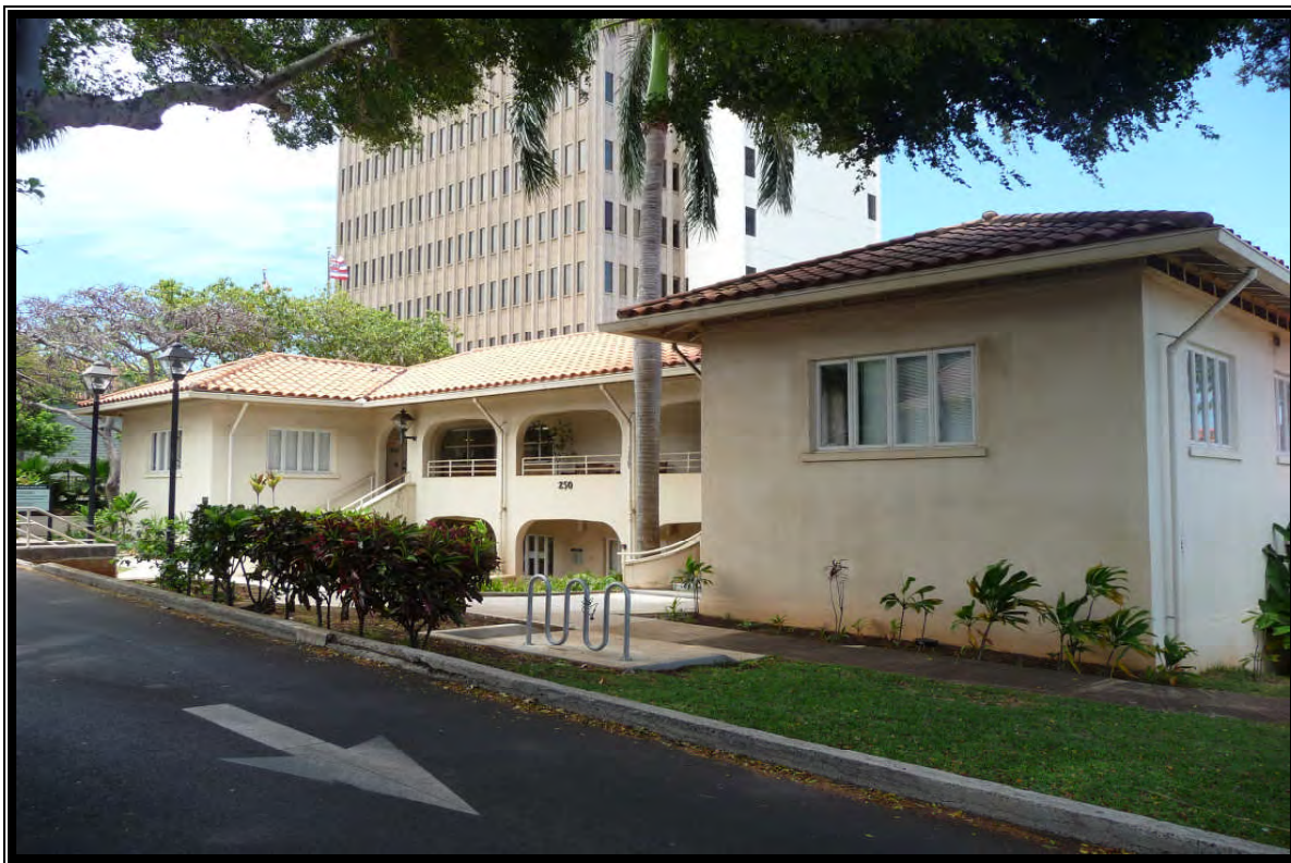
The renovated Kalana Pāku 'i Building, Wailuku.
