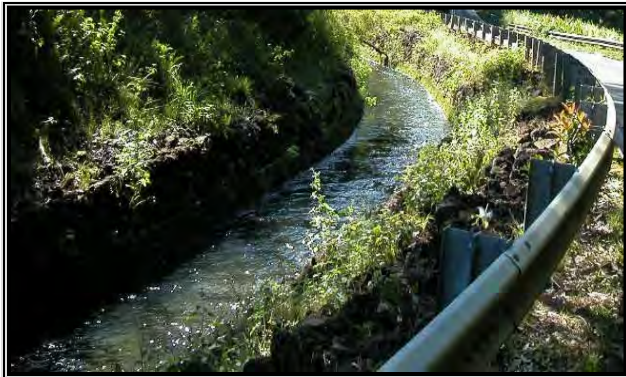
East Maui Irrigation Ditch.
